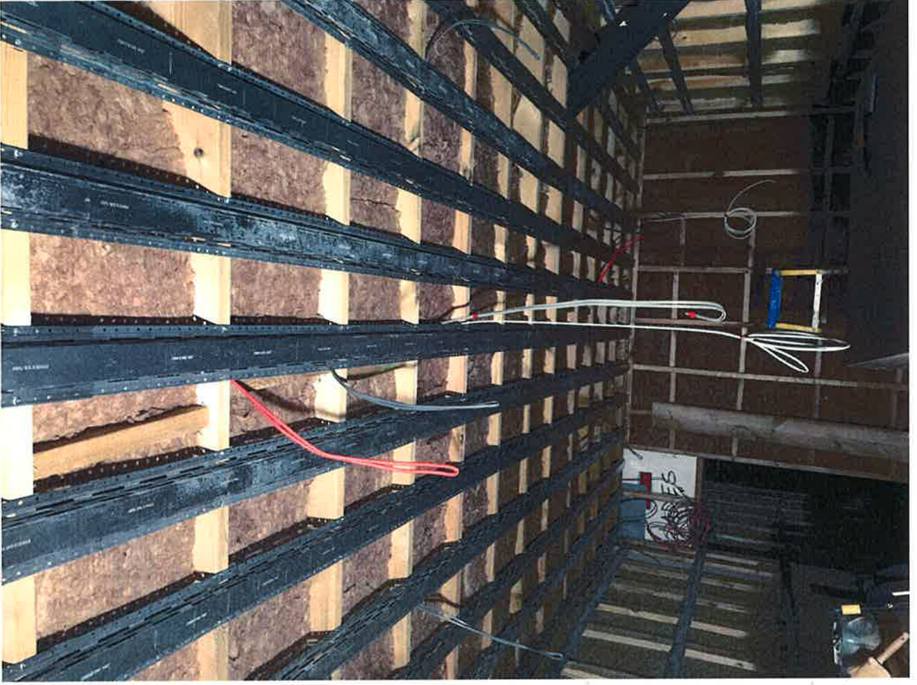
SOUNDPROOFING TO THE WALLS AND CEILING
