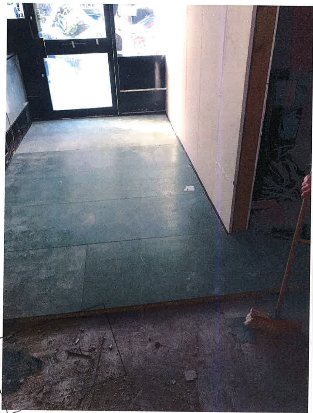
SOUNDPROOFING THE FLOOR.
